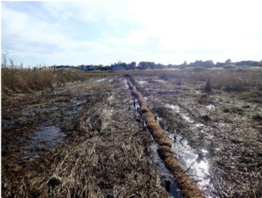
Left; Marsh surface prior to drainage channel and runnels, Right Surface after drainage channel and runnels installed, note all the new vegetation growing in previously flooded pannes. Bottom; Filling of ditches with coir logs and covered with marsh peat.
